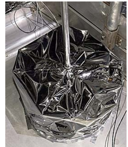
Closeout of Down Rods Source: Harris Corp.
